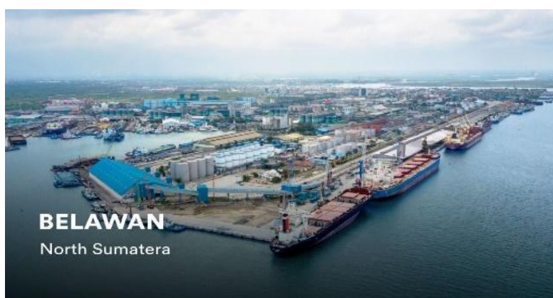
Gambar 1. Pelindo Multi Terminal
